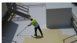
Also for Tenerife Airport the solution was Impermax 2K. It allows covering large surfaces in a minimum time.
